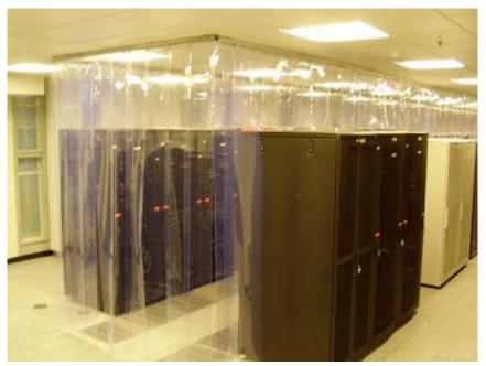
Use cold corridors (or home made cold corridor) to improve cooling efficiency by separating hot air and cold air.
